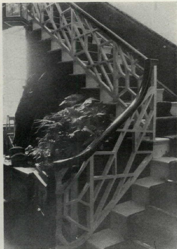
LOWER PART OF STAIRWAY
