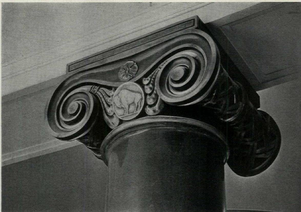
Marble Column in Main Banking Room
